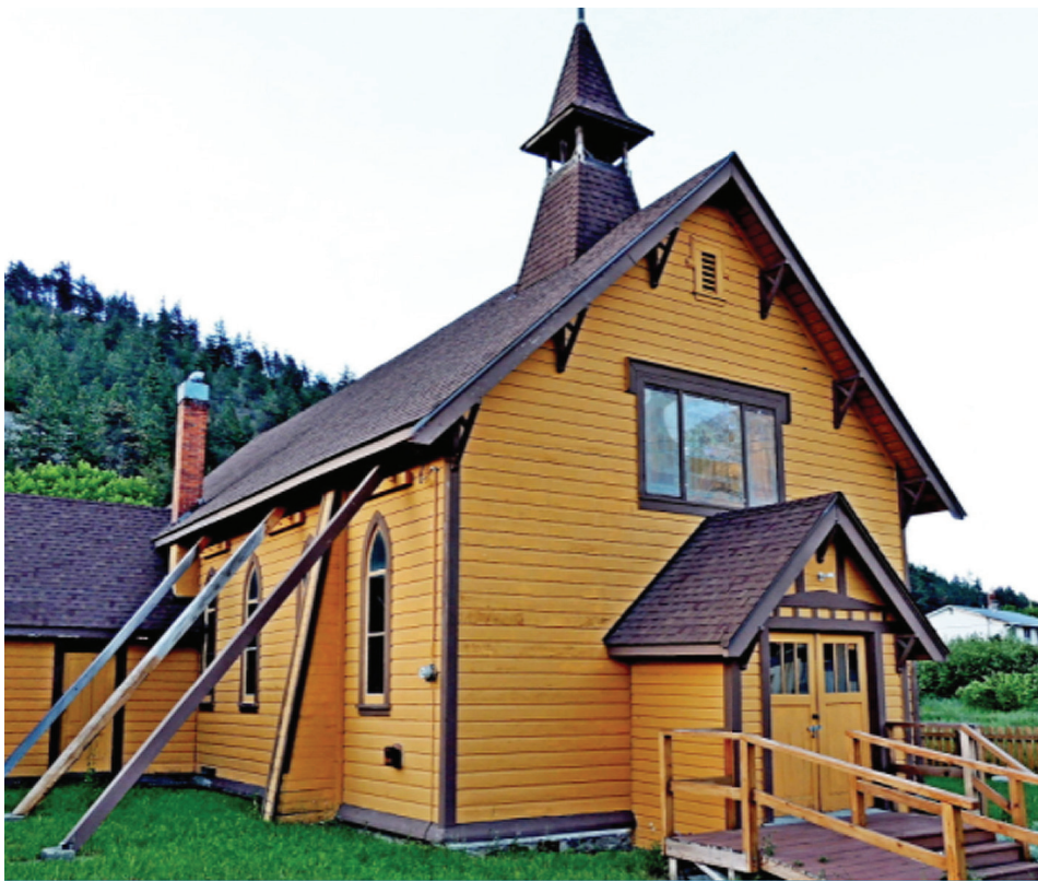
St. Mary and St. Paul Anglican Church, located on Lytton First Nation land, was totally destroyed in the fire.
