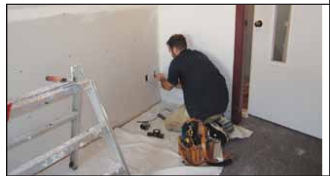
An electrician working on upgrading the electrical system
